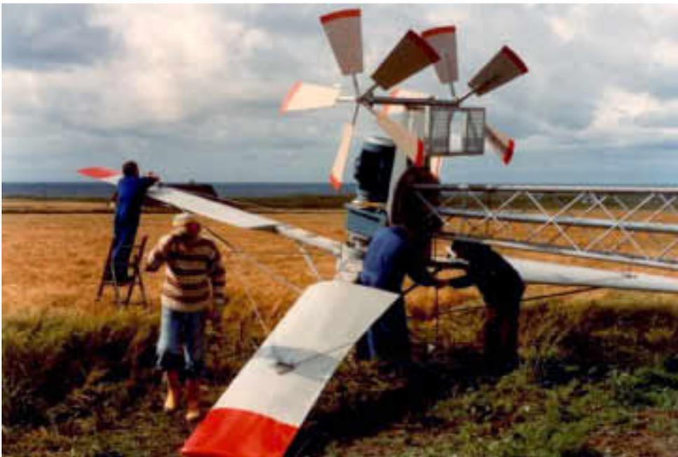
**Erecting a 30 kW Riisager wind turbine at Bovbjerg on the Danish North Sea coast 1978. The tail fan yaw mechanism is the same as used on the older Danish windmills.**
