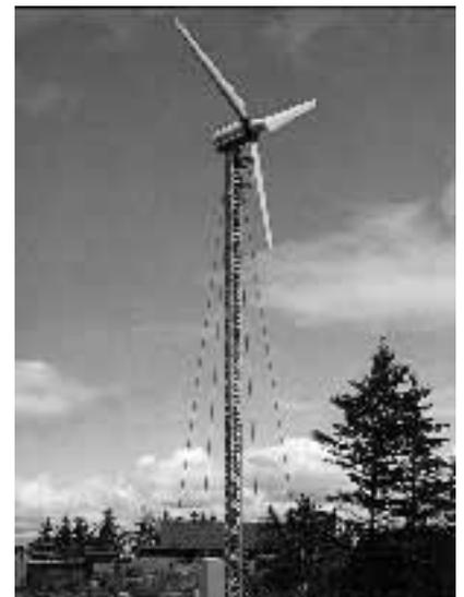
The “Kuriant” wind turbine (originally “Adolfsen”) was first to get the new “system certification” from Risø in August 1979 and it was in the following years a close competitor to the Riisager turbines. With its downwind placed rotor (like the Tvind turbines) it was different from most other Danish wind turbines.
