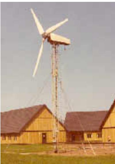
The small “PTG-turbine” built by the Tvind schools in 1978 used the same blade construction as the big wind turbine. Its design was a starting point for a new Danish blade concept. (Photo: Erik Grove-Nielsen)
